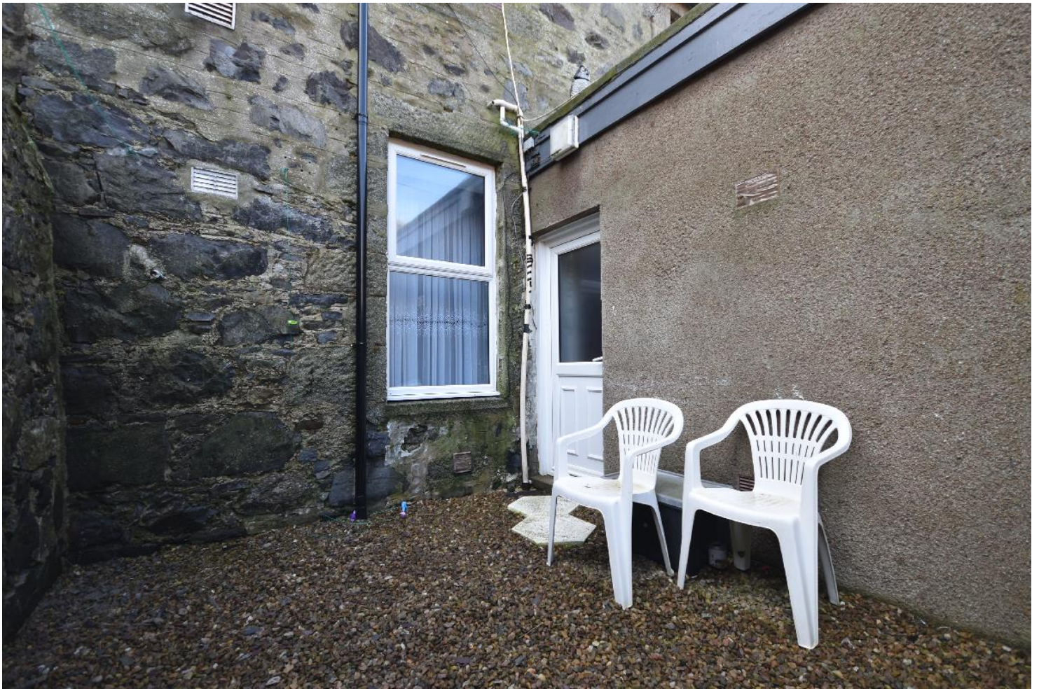
REAR COURTYARD ALTERNATIVE VIEW
